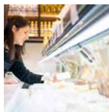
Refrigerated units and cold rooms
